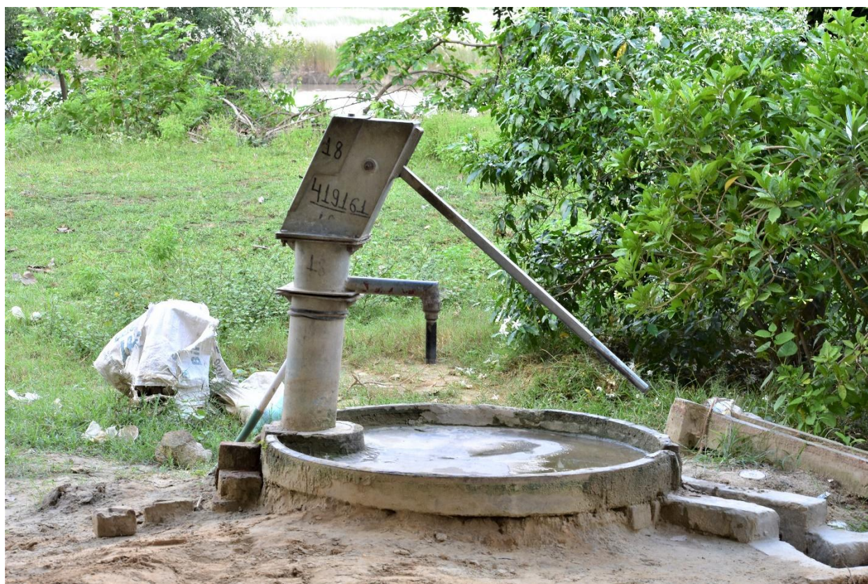
Image 40 : Hand pumps Used For Ground Water Extraction In Study Region
